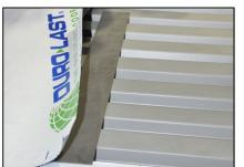
4. On steel decks, at the end of a roll, install a metal plate (6 in. by 42 in.) to support the vapor barrier end lap between the metal flutes ensuring a complete end lap seal. End laps must overlap by 6 inches.
