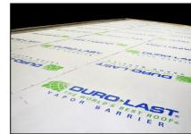
6. Once installation is complete, the Duro-Last Vapor Barrier temporarily protects against inclement weather. If not immediately covered, follow extra steps per 3a and 3b in the instructions above.
