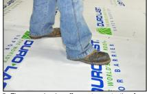
5. The vapor barrier offers extra protection from heavy foot traffic during installation. The slipresistant surface allows for safe movement across the roof.
