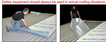
1. Roll out the Duro-Last Vapor Barrier over a clean, drv deck
