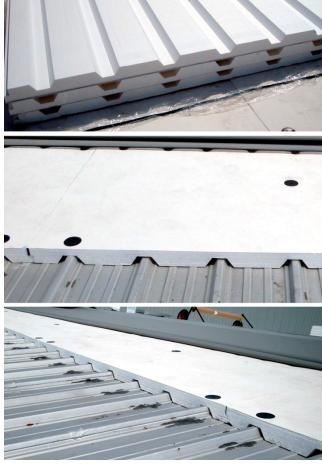
Figure 1. Duro-Guard EPS Flute Fill Combo with FR facer
