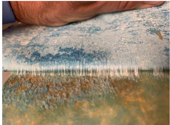
Acceptable Duro-Last Solvent-Grip “legging/stringing”
