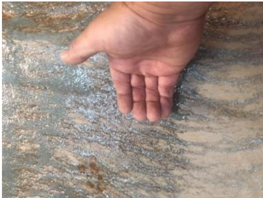
Checking for dry Duro-Last Solvent-Grip
