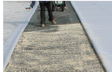
Figure 2. Applying Adhesive in Splatter Pattern
